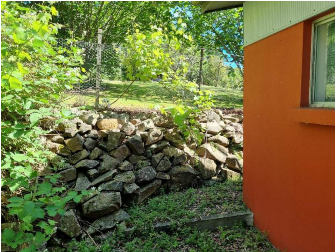
Photo 4: Dry-stacked dolerite boulder retaining wall adjacent to existing dwelling, looking north.
