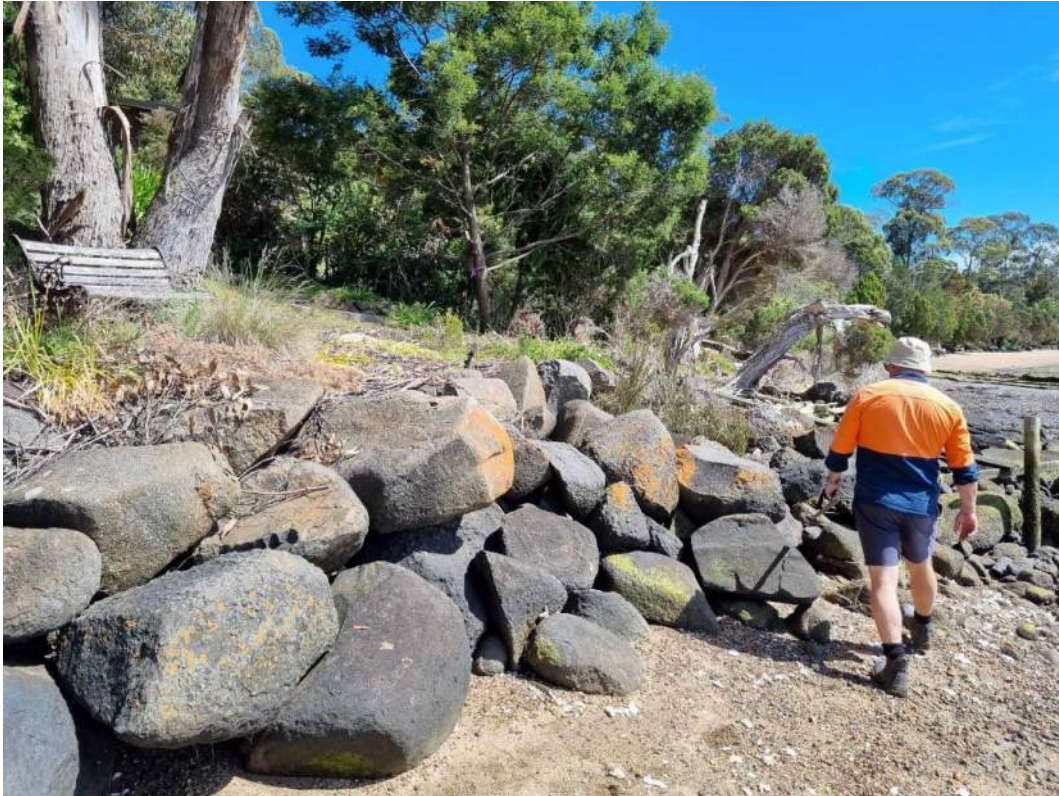
Photo 9: Dry-stacked dolerite boulder wall on eastern boundary of site to protect site from erosion.
