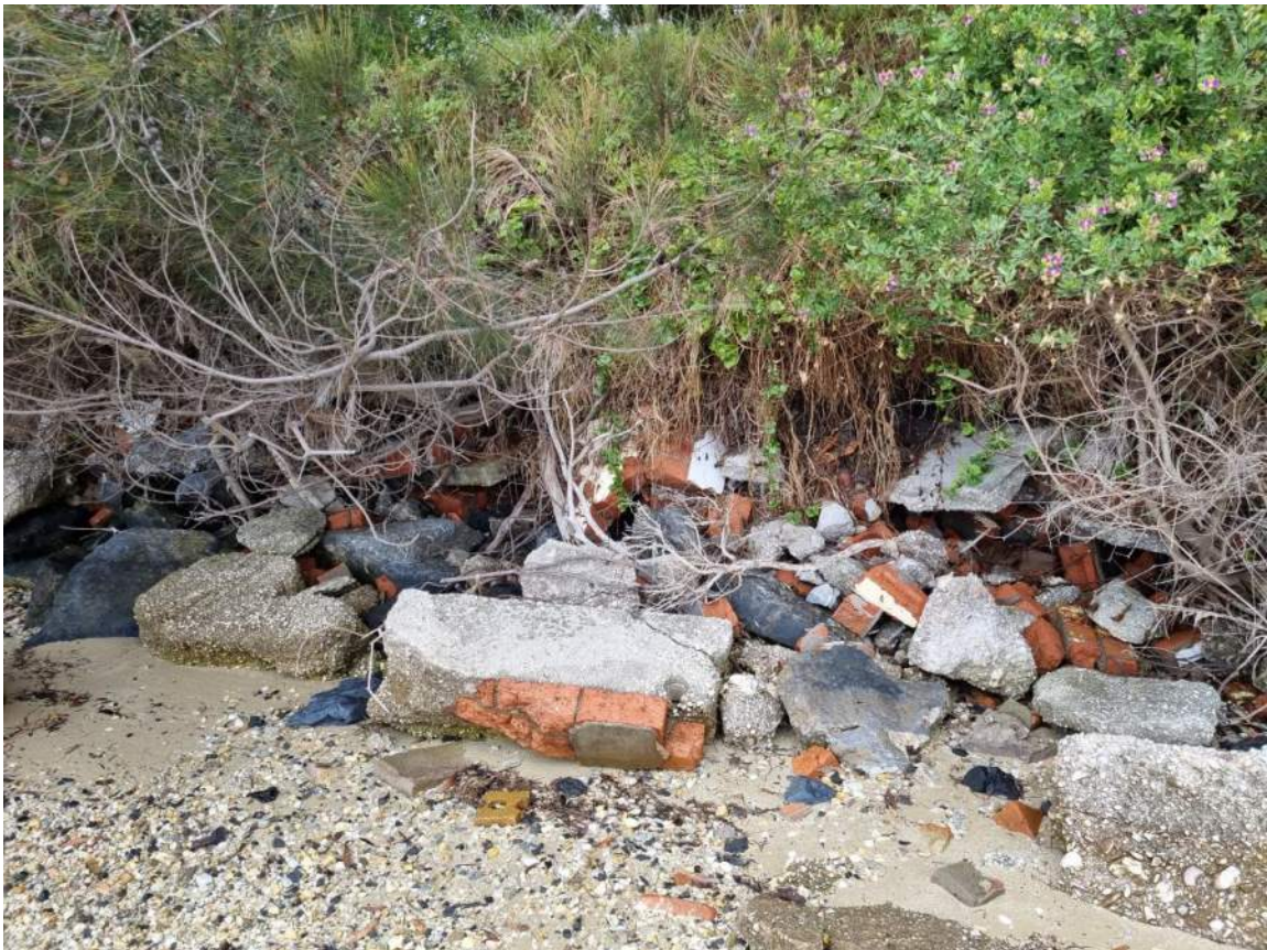
Photo 10. Makeshift erosion protection on western shoreline.
