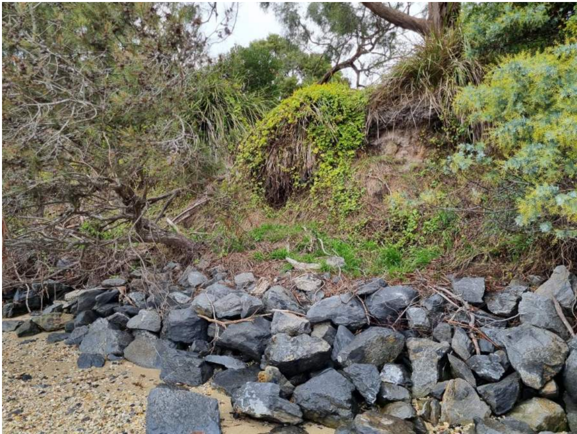
Photo 11. Erosion protection at toe of ~2m high scarp on western shore.
