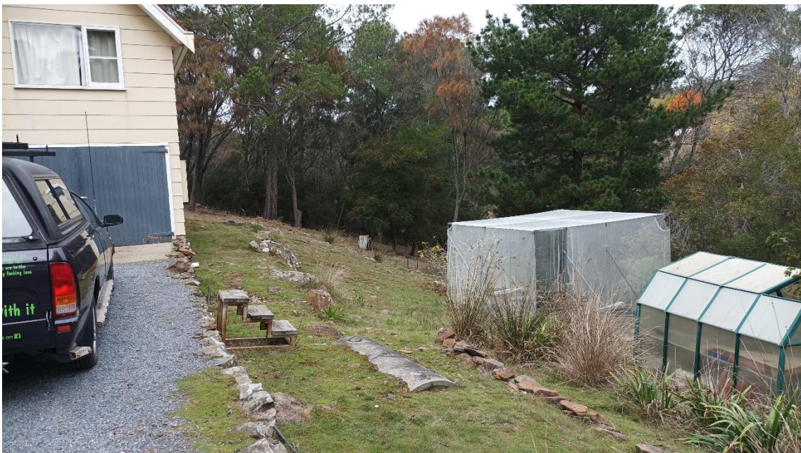
Plate 2: View of the existing septic tank looking to the south 20/05/2025.
