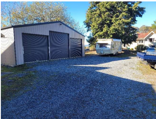
Figure 10 existing access at the dwelling in lot 2.
