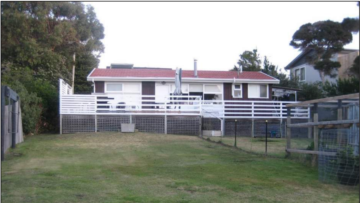
Figure 4: Image of northern elevation of existing dwelling (photo taken 10/08/2025).
