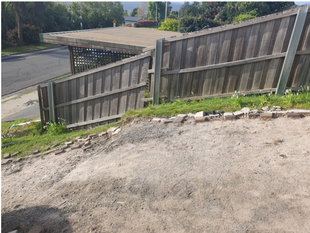
PLATE 2 - View of landslide headscarp displacement through driveway and fence
