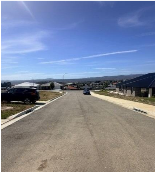
Figure 3: Faye Court Facing East
