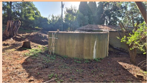
Existing concrete tank – Lot 1 (appears to be domestic supply)
