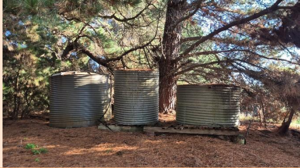
Existing tanks – Lot 1
