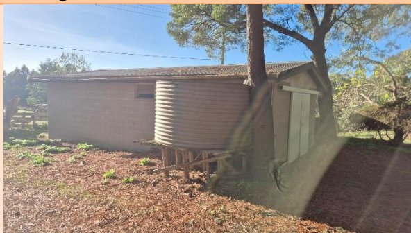
Existing small metal tank – Lot 1
