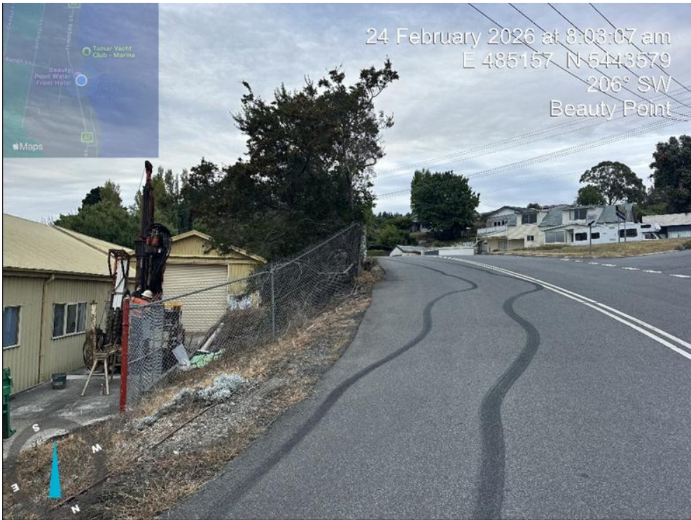
Plate 2: View of Flinders Street and existing driveway during Borehole BH2 drilling.
