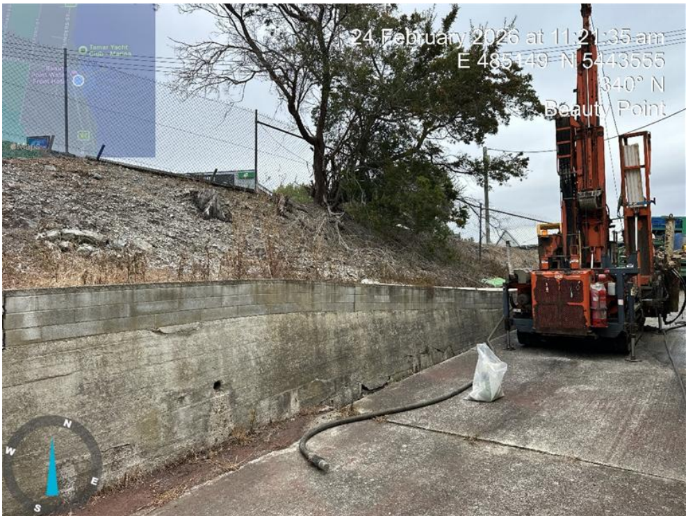
Plate 1: View of the site during Borehole BH2 drilling, showing the existing driveway and retaining wall (to be replaced), looking towards northwest, 24.02.2026.
