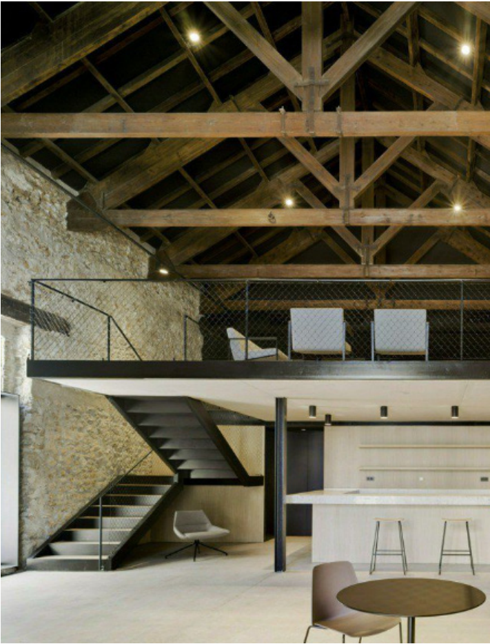
Ceiling: Exposed trusses
