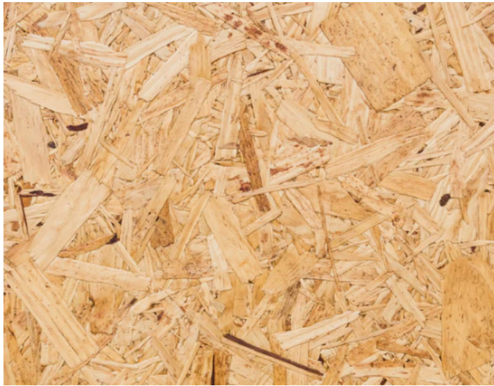
WORKSHOP A - CEILING: OSB
