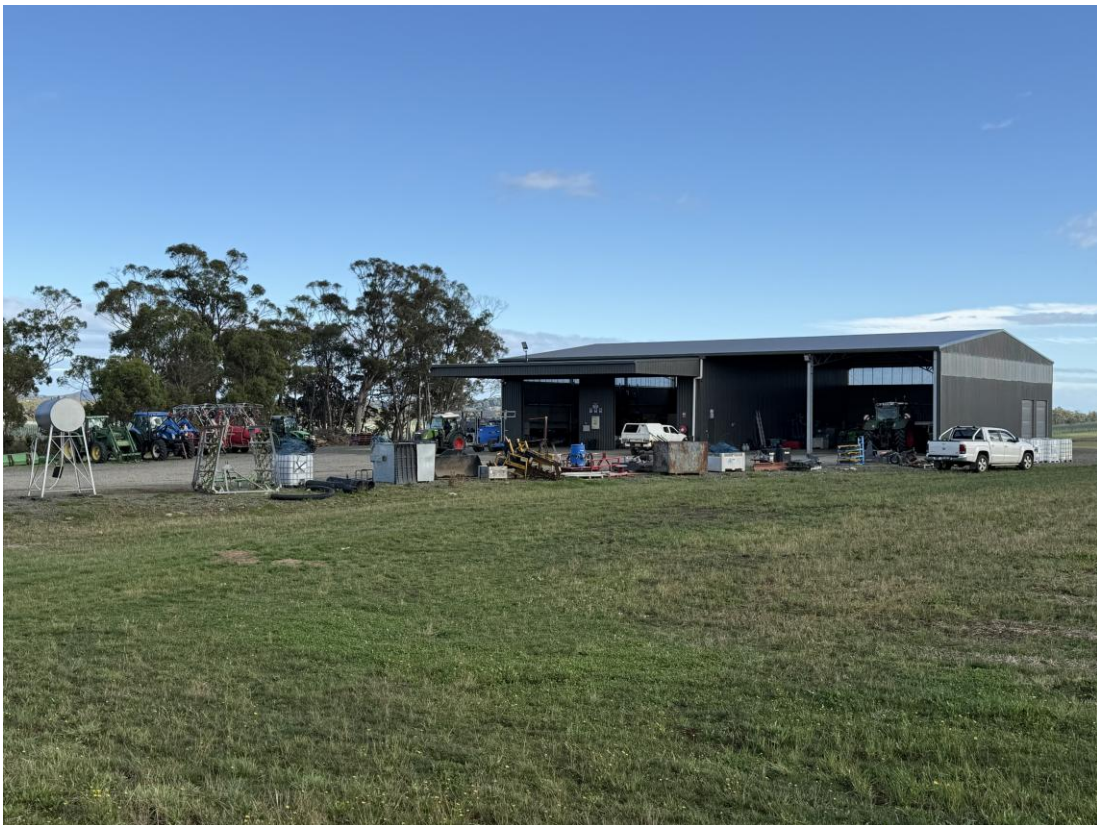
Image 12 View of the machinery shed located to the immediate north of the irrigation dam present, as would be located on the proposed Lot 1. Taken at site assessment 26/3/2026.
