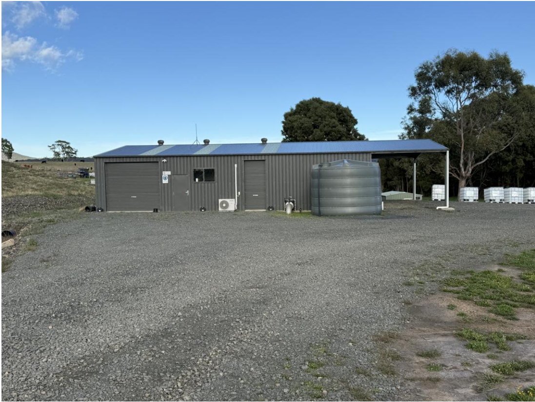
Image 11 View of the pump shed located to the immediate north of the irrigation dam present, as would be located on the proposed Lot 1. Taken at site assessment 26/3/2026.
