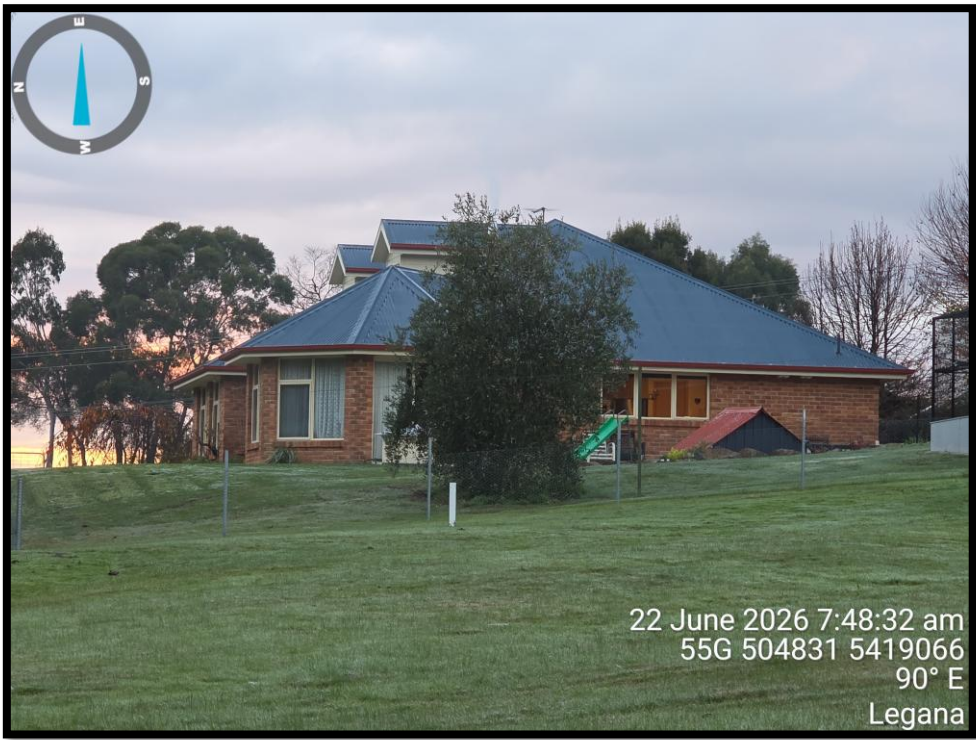
Plate 1: View of the existing dwelling looking to the east.
