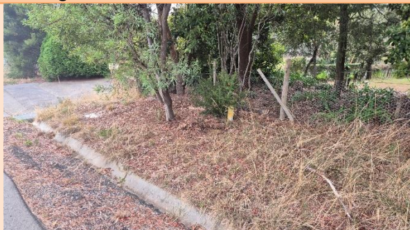
Existing fire plug to northeast
