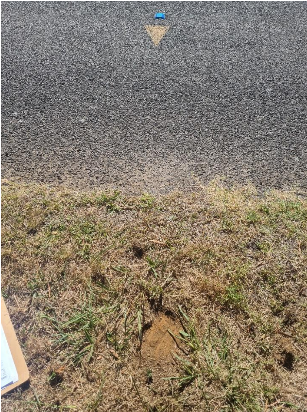
Image 5.1 – Hydrant located northwest on Upper McEwans Road
