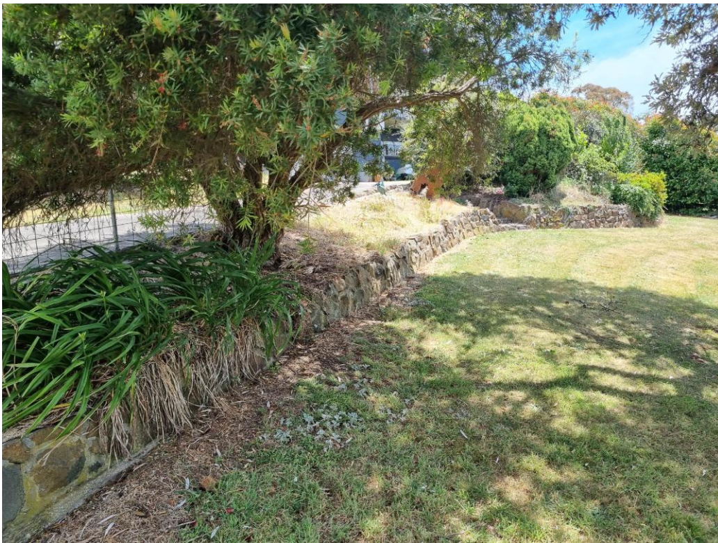
Photo 10. Cobble/boulder and concrete landscape retaining wall in front yard of existing dwelling, looking northwest.
