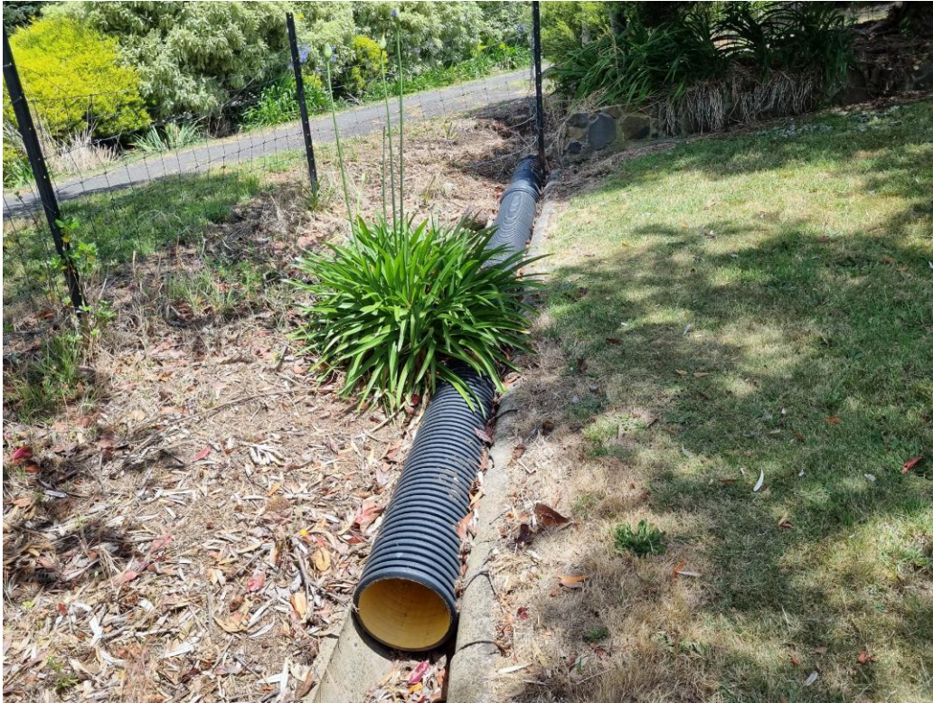
Photo 11. Culvert under existing driveway and concrete spoon drain, looking southwest.
