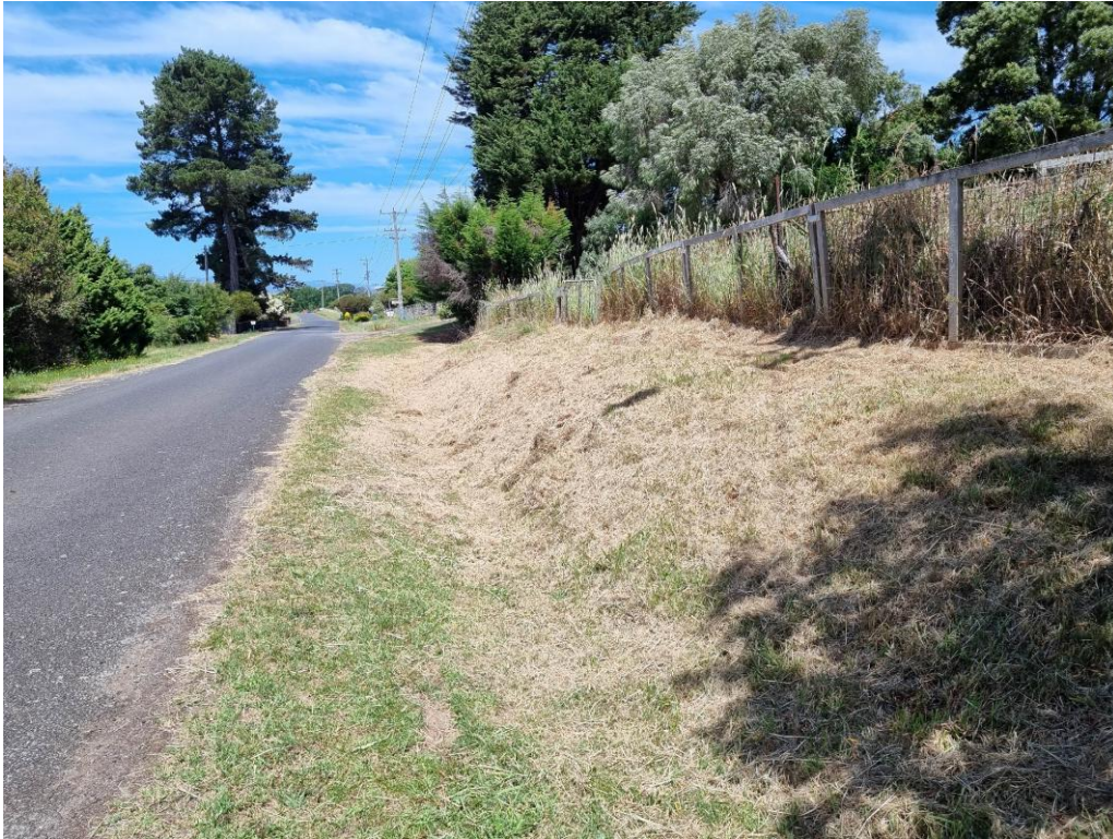
Photo 3. Cut slope up to ~0.7m high on between Upper McEwans Road and northeastern boundary of site, looking southeast.
