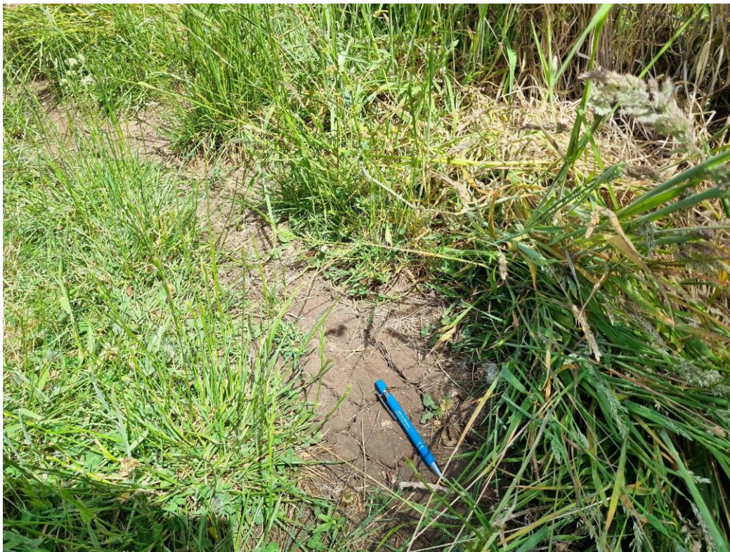
Photo 20. Desiccation cracking in surface soils on proposed Lot 2.
