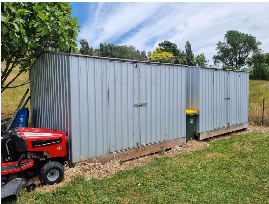
Photo 5. Existing aluminium sheds looking ~west.
